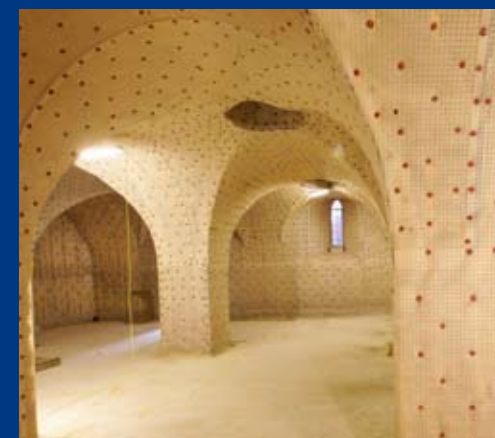
Newton Membranes can be used to deal with all types of damp including rising and penetrating damp
