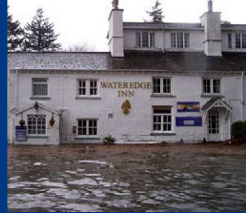
High levels of rainfall in the UK causes many damp problems
